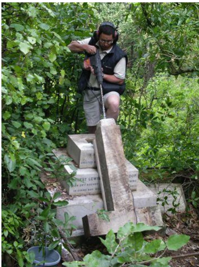
Repair of the Widdop memorial (grid F10-1) on Trustees Crescent path.
