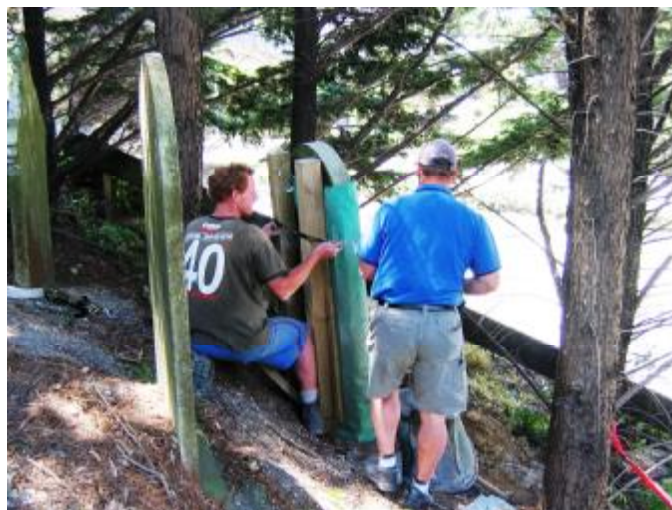
Contractors prepare to move Turnbull memorial, 5 Dec 07. Photo Kate Fortune
