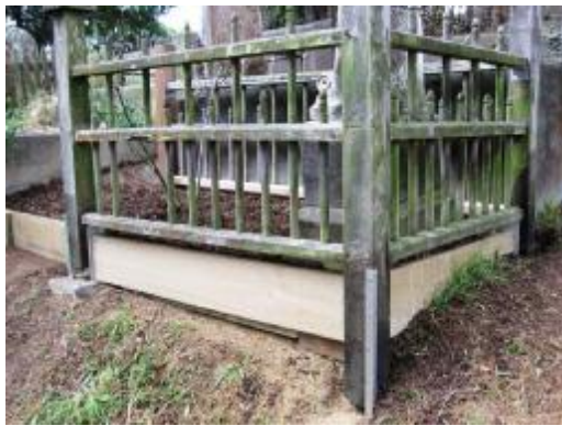
Laurie grave repaired
