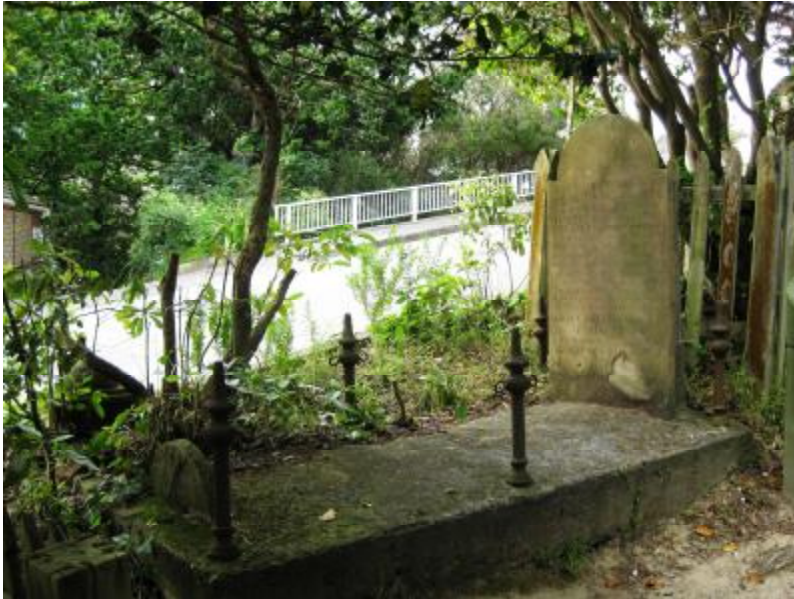
Gillespie grave in 2010, showing delamination and buried head and foot stones. Photo: Kate Fortune
